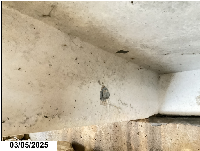
Span 2 bent 3 unit 2 left leg has a hairline to minor sized shear crack through bolted connection.
