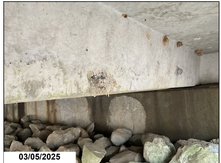
Span 1 Bent 1 Unit 1 right leg small spall with exposed rebar.
