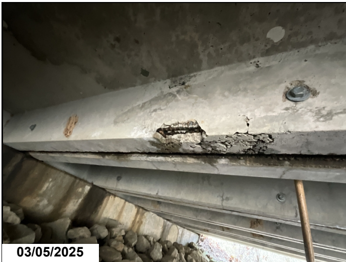
Span 1 Bent 1 Unit 6 left leg has a 2' honeycomb area exposing 1' of rebar
