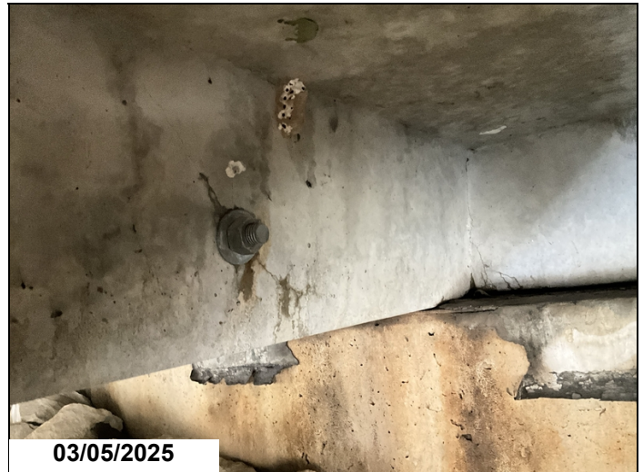
Span 2 Bent 3 Unit 4 left leg has a shear crack through bolted connection.
