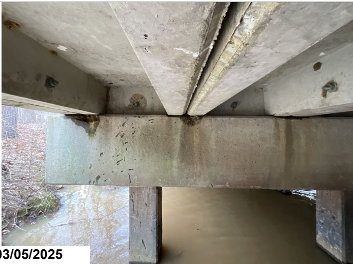
Bent 2 back side typical of spalls under units
