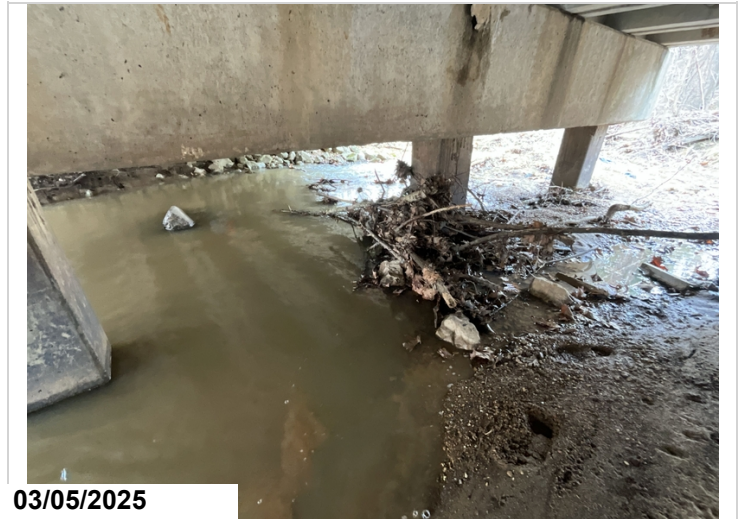
Bent 2 pile 3 minor drift buildup
